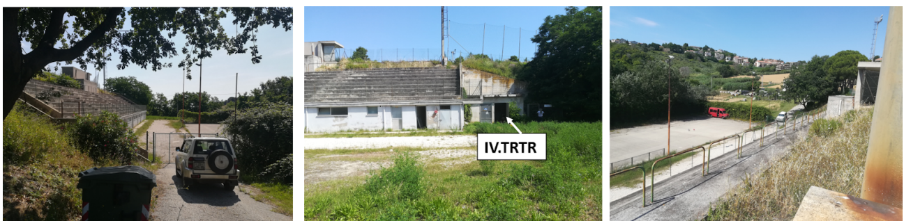
Figure 2. Pictures showing the driveway (left); the cabinet housing IV.TRTR and the bleacher of the stadium (middle); the driveway and the concrete square are seen from the level of the uppermost football field (right).
