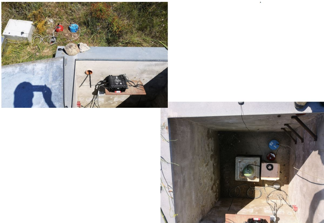
Figure 7: A Reftek130 connected to Le3d5s together with a Terrabot were situated at the surface (on the left) and at the bottom (on the right) of the inspection pit. Measurements were carried out on the 31th of July 2019.
